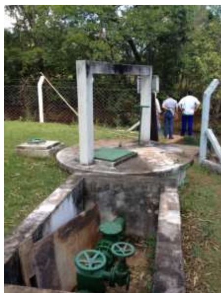
Barrilete de Recalque
