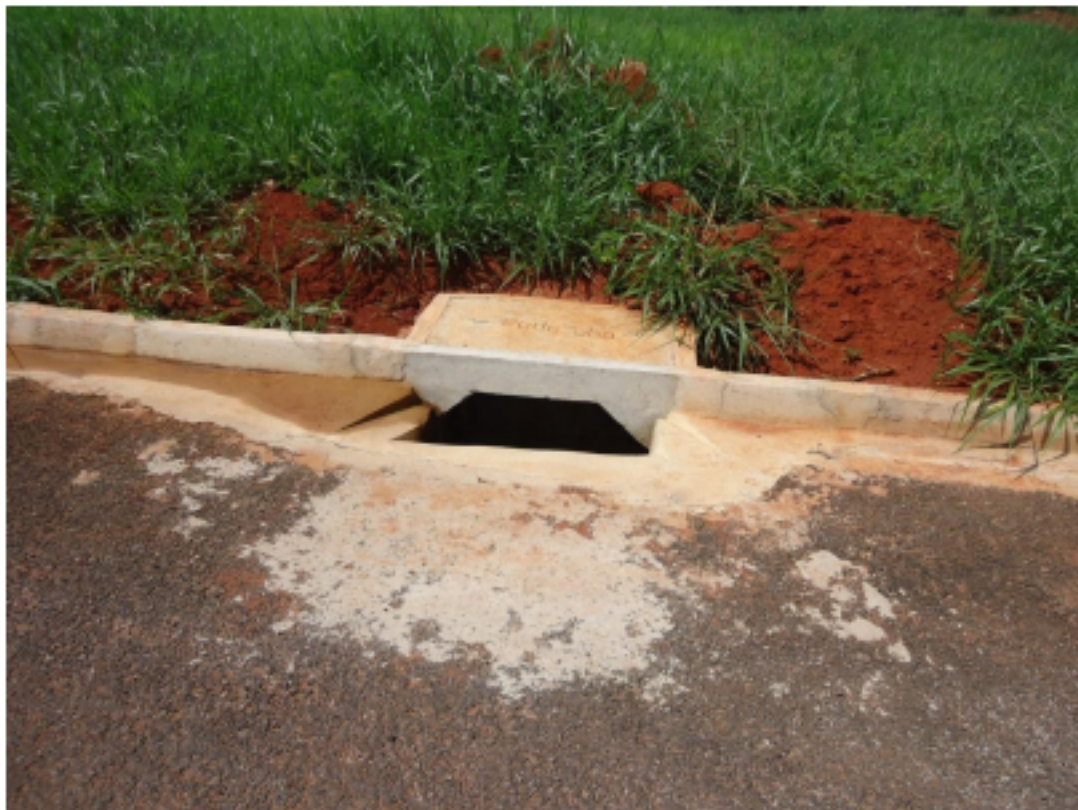
Figura 41 –Galeria Pluvial Residencial Zizinha
